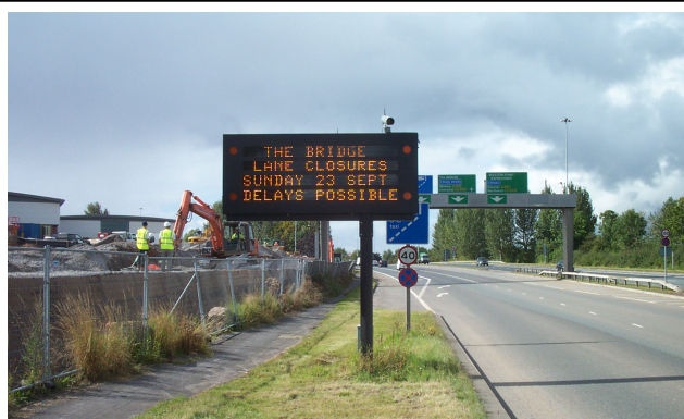
VMS with ANPR camera, Bridgewater Expressway
